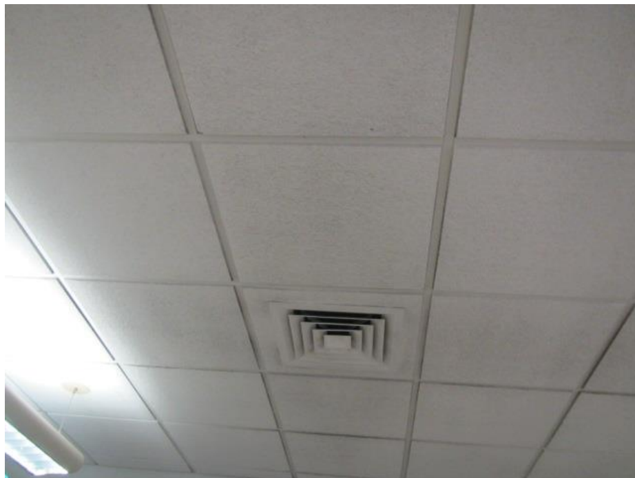
Ceiling-mounted supply diffuser
