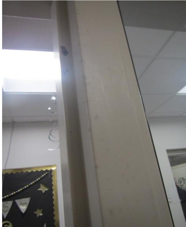
Mold growth (spotting) on metal door jambs in Guidance Suite
