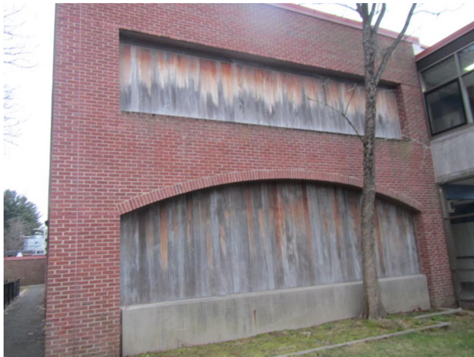
Delaminating paint/stain exposing wood covering windows in original 1969 portion of building, also note close proximity of tree to foundation/exterior wall
