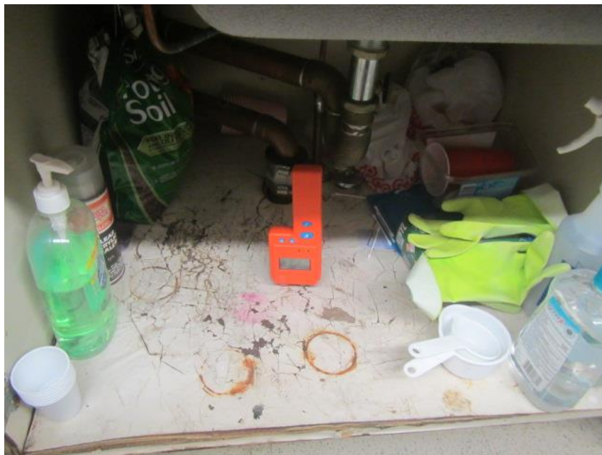
Water-damaged particle board under classroom sink Note: moisture meter indicating wood was dry at time of assessment
