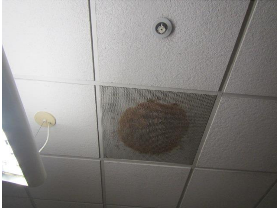
Ceiling-mounted return vent in classroom, note corrosion/staining
