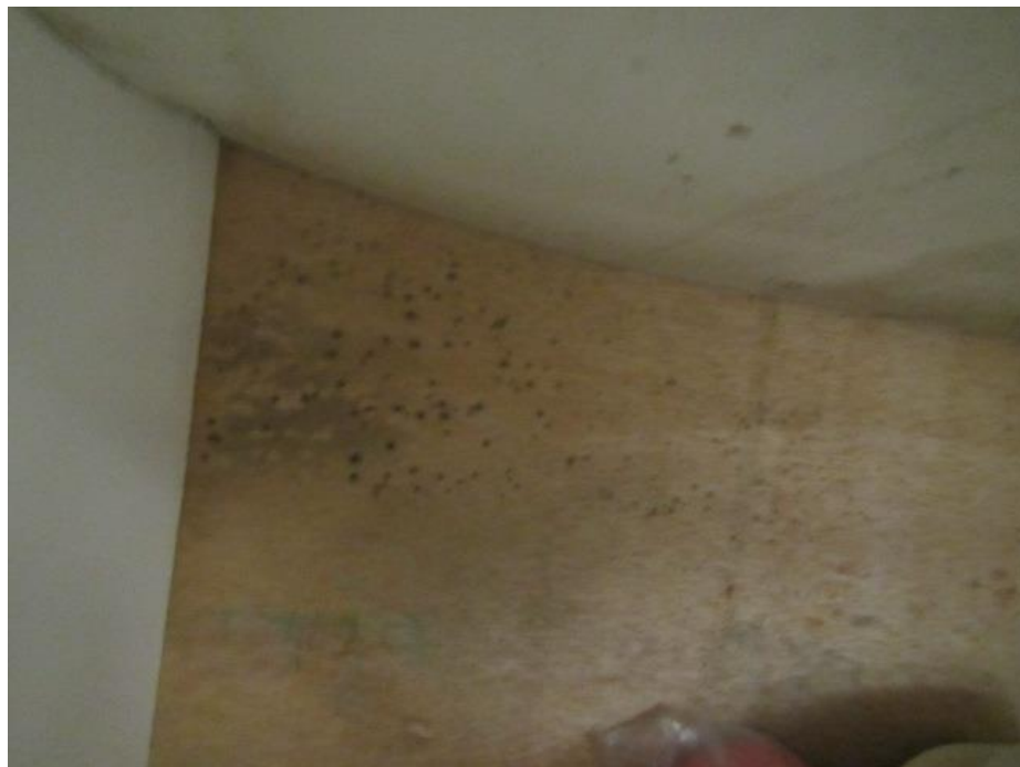
Small dark spots indicate likely mold on plywood cabinet in Room 107
