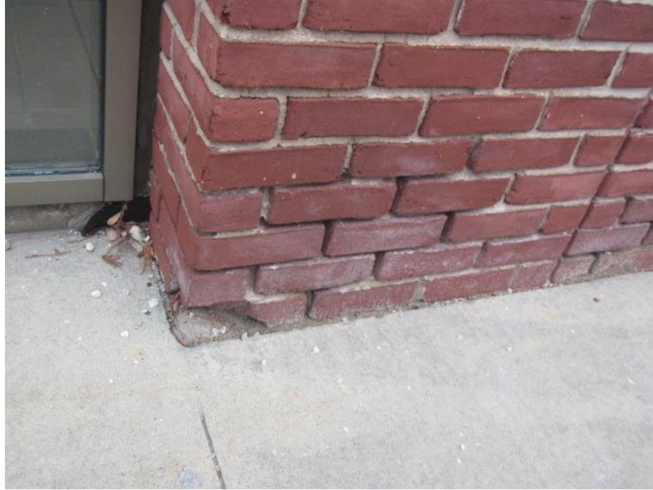
Missing/damaged mortar around exterior brick
