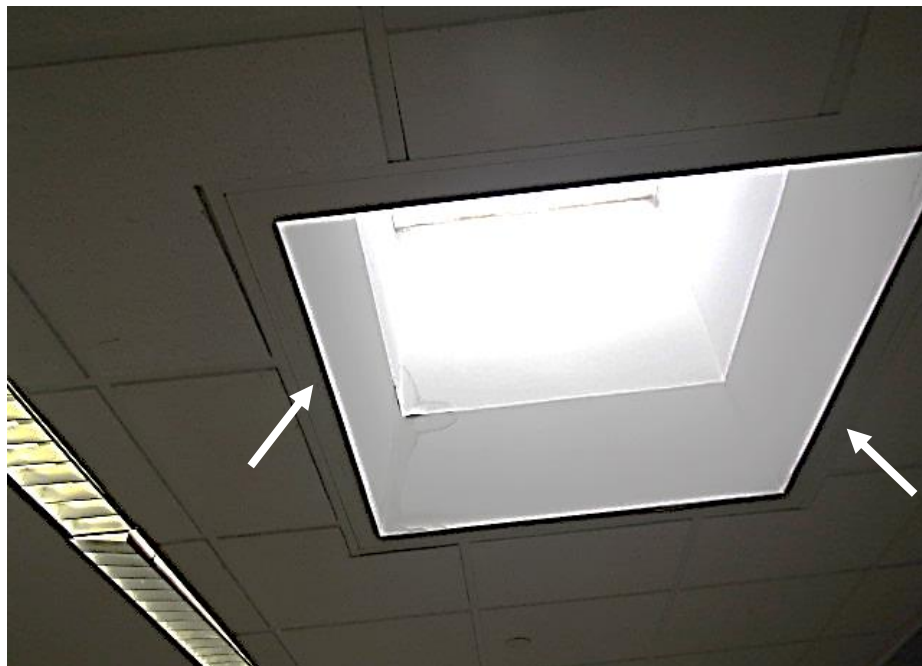
Water-damaged gypsum wallboard around skylight Note: light mold growth was noted on the surface around skylight (arrows)
