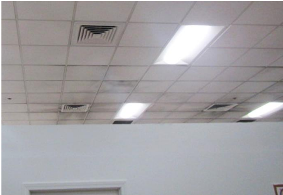
Accumulated dust and debris on vents and surrounding ceiling tiles
