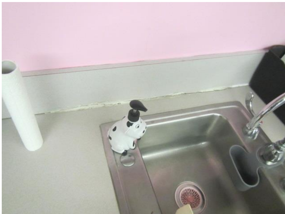
Missing/damaged caulking around classroom sink
