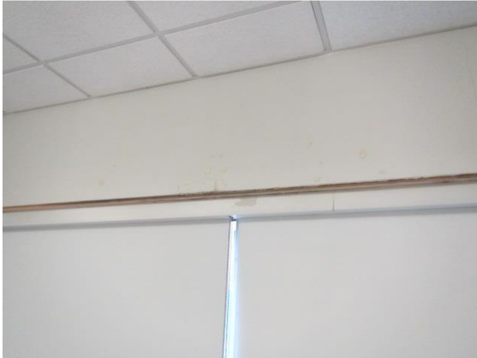
Water-damaged gypsum wallboard above windows in Room 216
