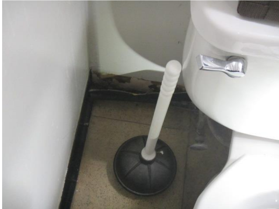
Visible mold observed behind coving in the restroom outside the Media Center
