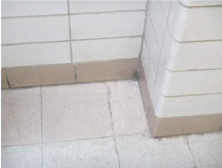
Area of water infiltration in hallway outside of Room 143
