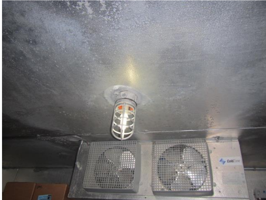
Condensation on ceiling of walk-in freezer
