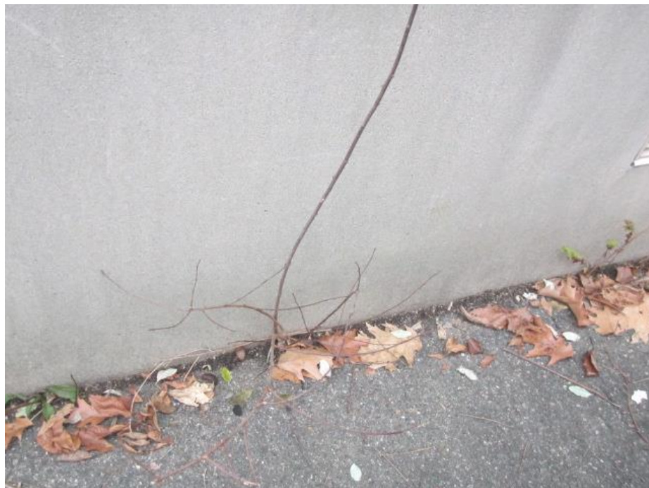
Plant growth along seam of concrete foundation and tarmac
