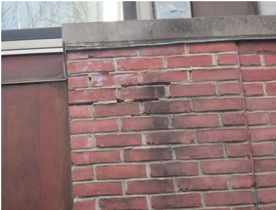
Missing/damaged mortar around exterior brick
