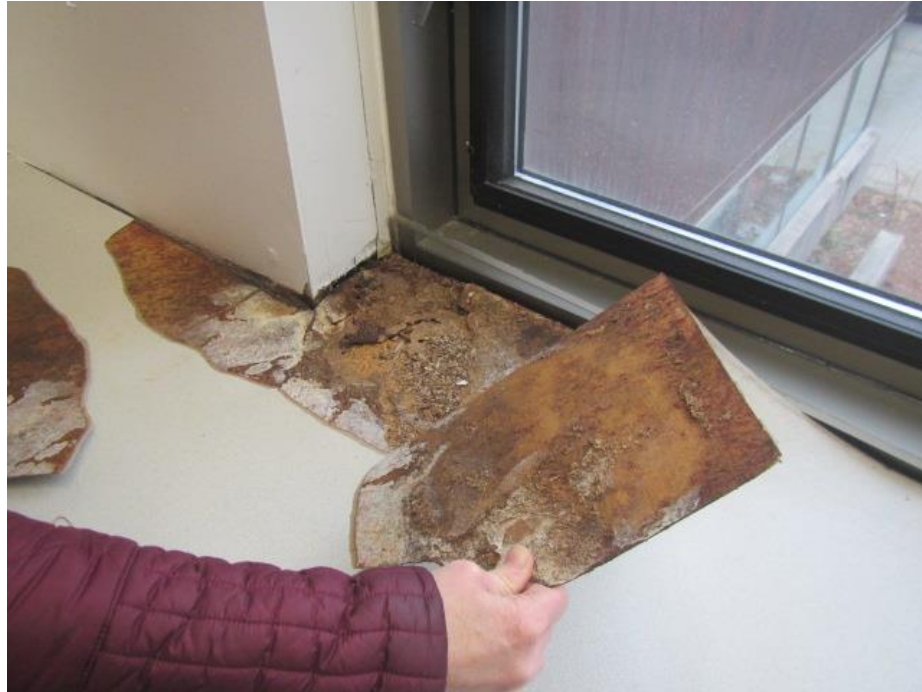
Water-damaged surfaces near windows in Media Center
