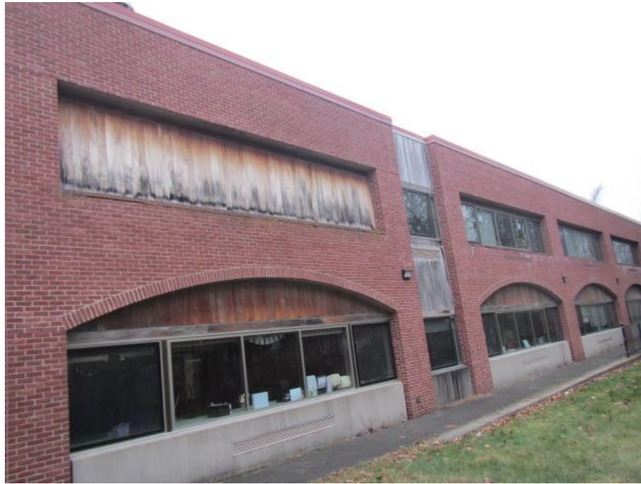
Delaminating paint/stain exposing wood covering windows in original 1969 portion of building
